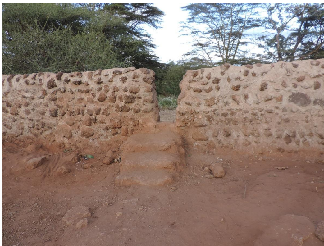
Figure 13. Photograph of the protective wall around the spring in Namelok which prevents contamination through livestock and wild animals
